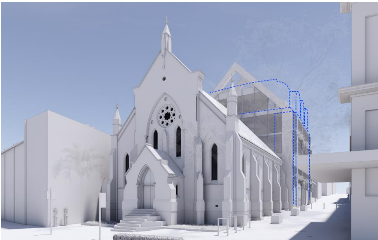
Figure 37: Render of proposed development from Cleveland Street with the approved form of the consented scheme (D/2020/993) dotted in blue
