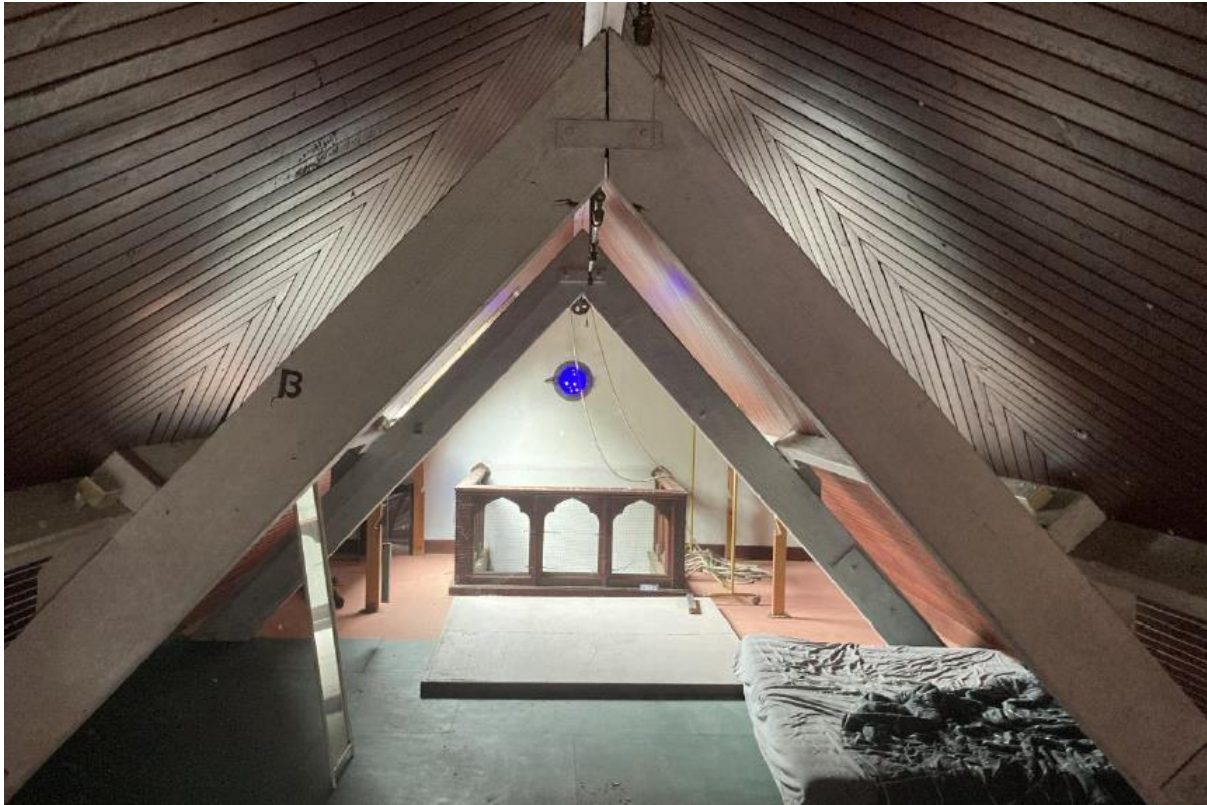
Figure 13: Internal of mezzanine level within existing church building
