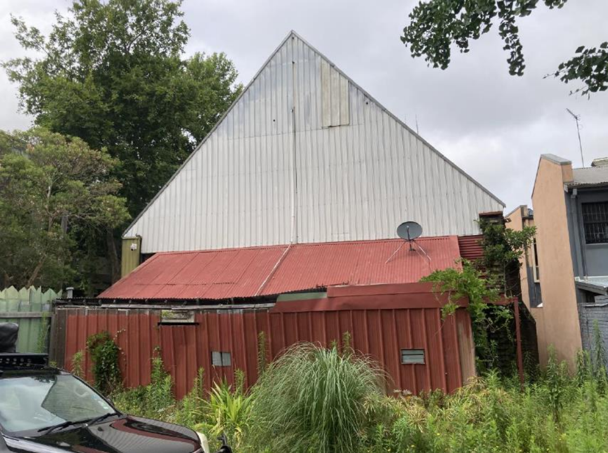
Figure 7: Rear of existing building viewed from rear setback looking south
