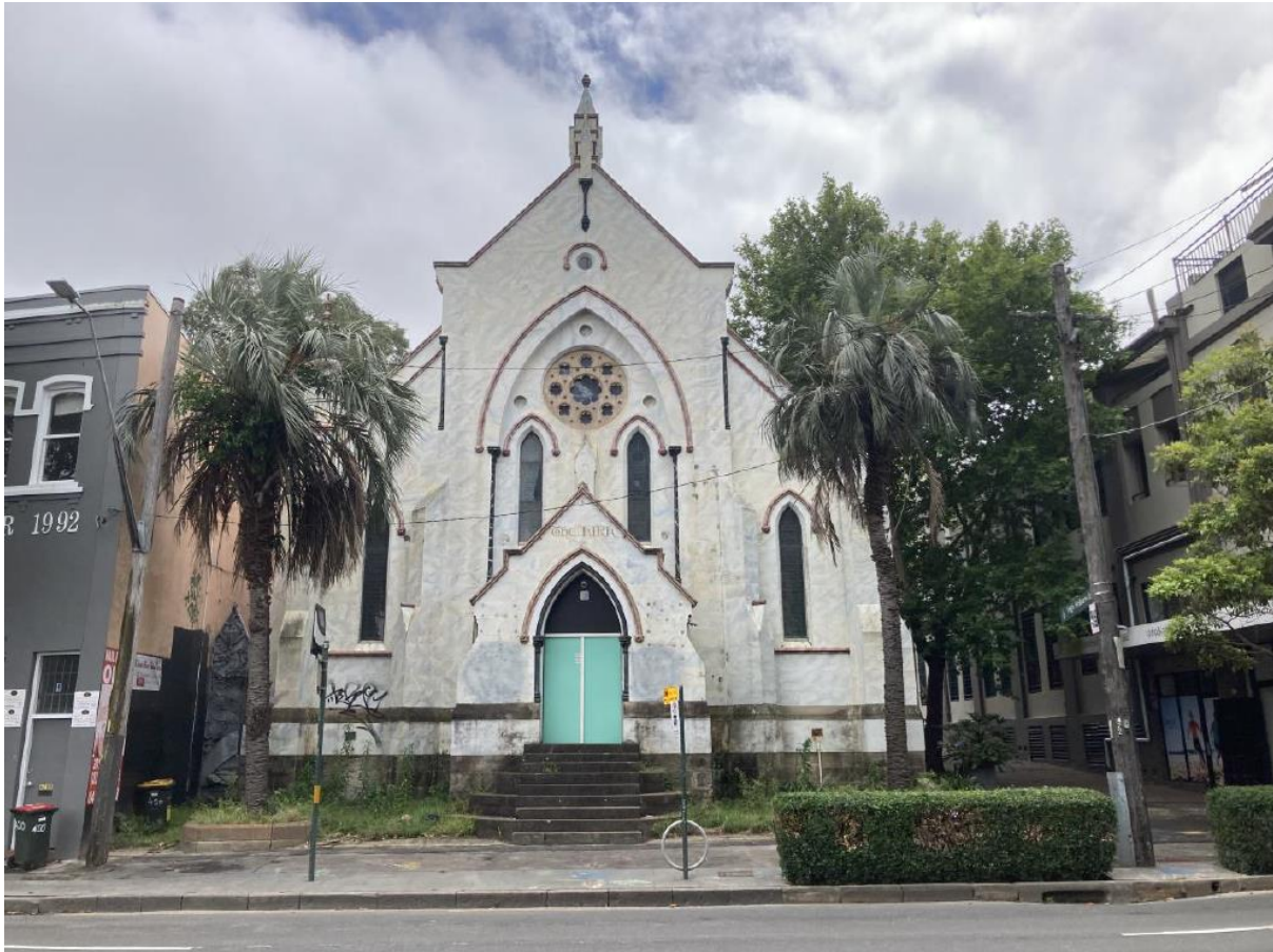
Figure 2: Front of site viewed from Cleveland Street looking north
