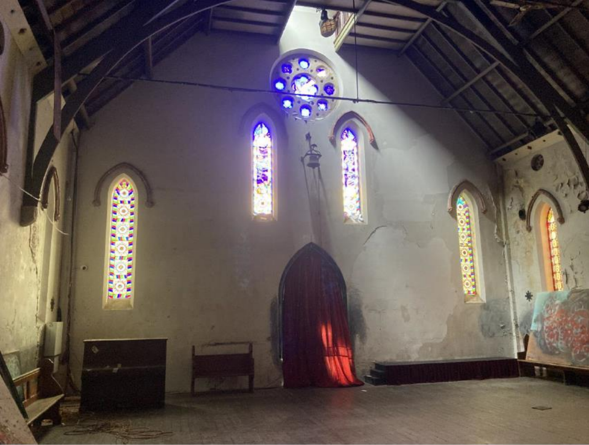
Figure 11: Internal of existing church hall
