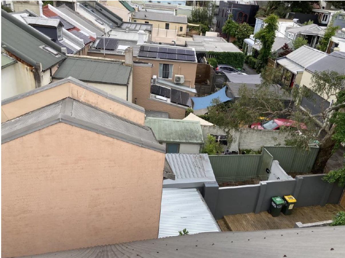
Figure 10: Rear of existing terraces backing on to the south side of Goodlet Lane, viewed from the mezzanine level of the existing church building looking west
